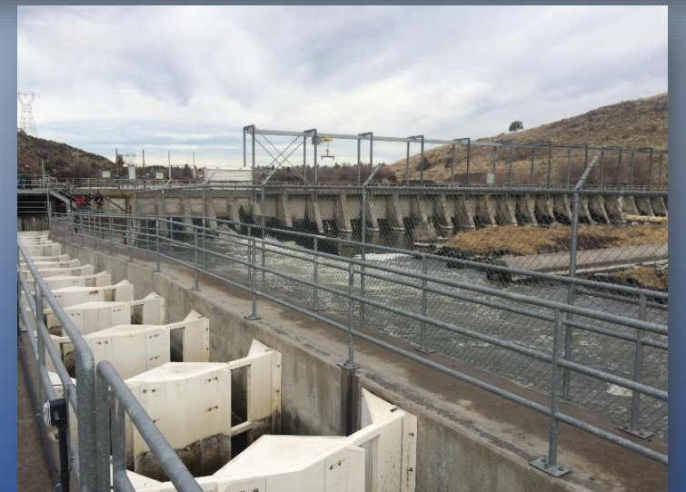
Link River Dam (outlet of Upper Klamath Lake)
